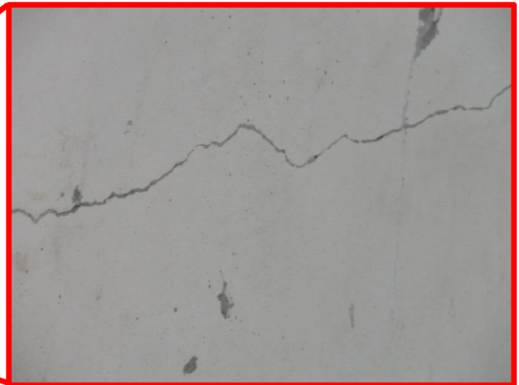
Crack in wall panel
