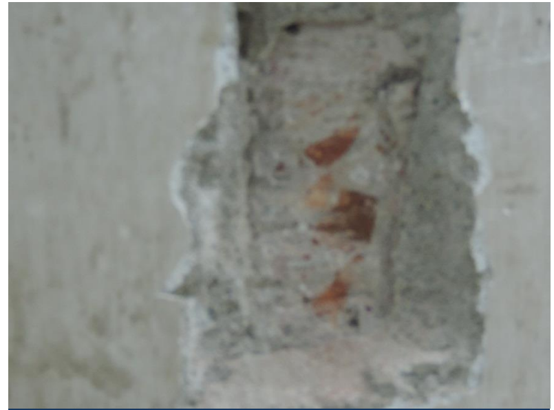
Brick aggregate in column
