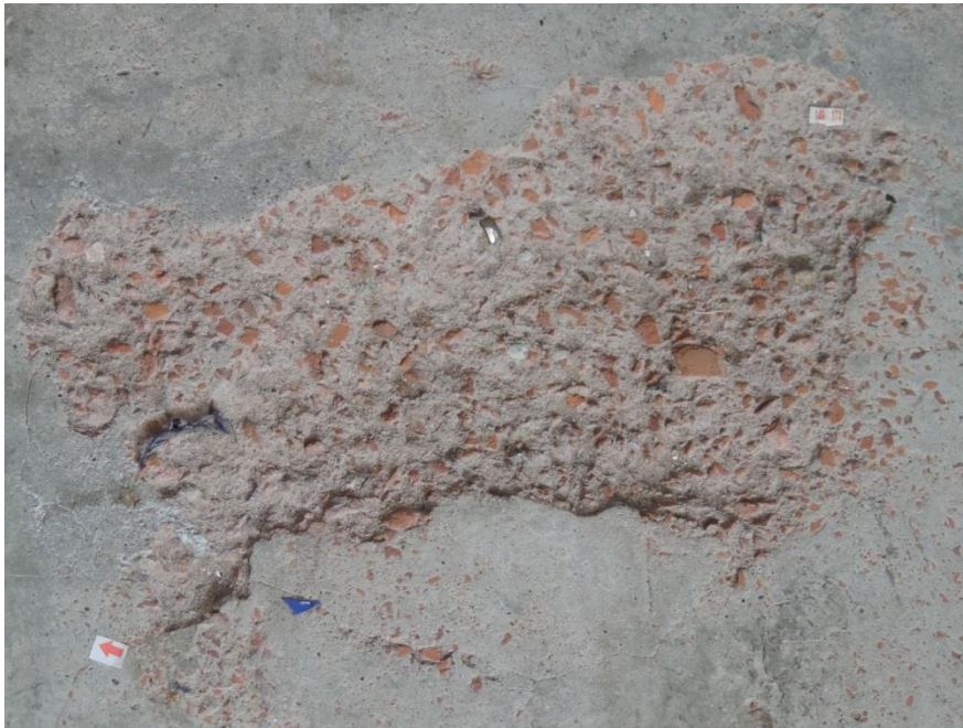
Brick aggregate in slab
