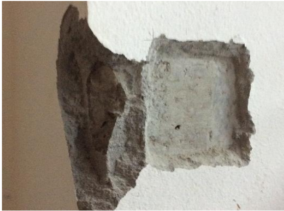
Tested Column showing brick aggregate.
