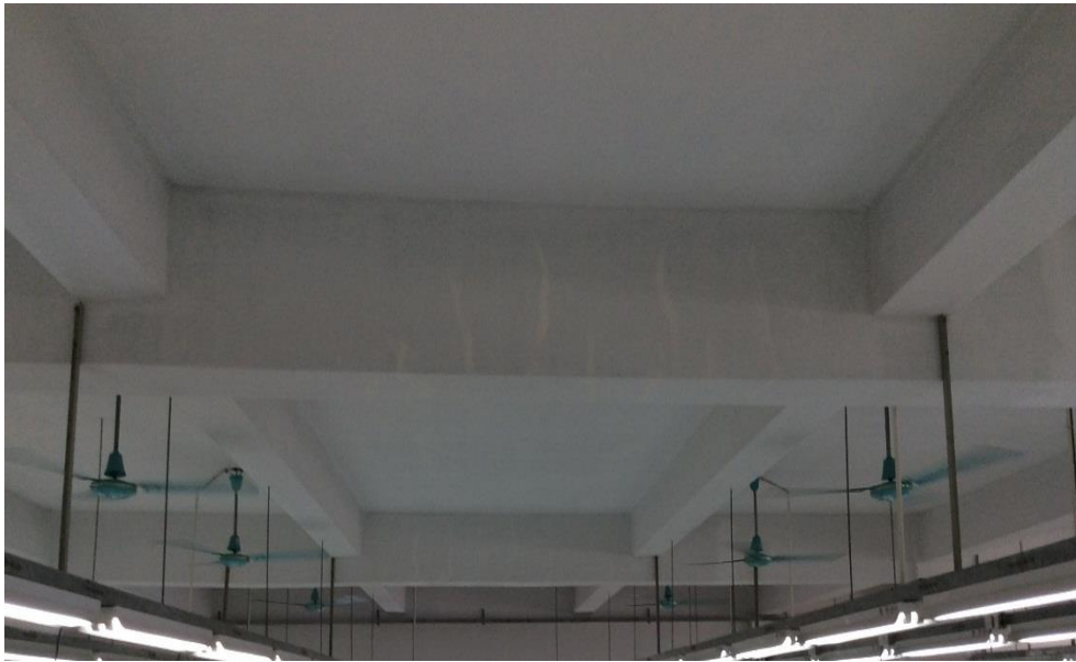
Cracks Repaired to side of the beam
