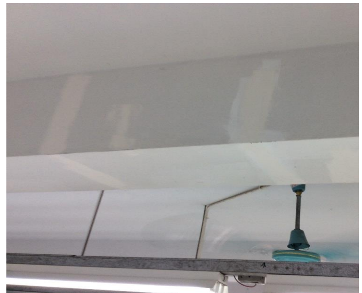
Cracks Repaired to underside and side of the beam
