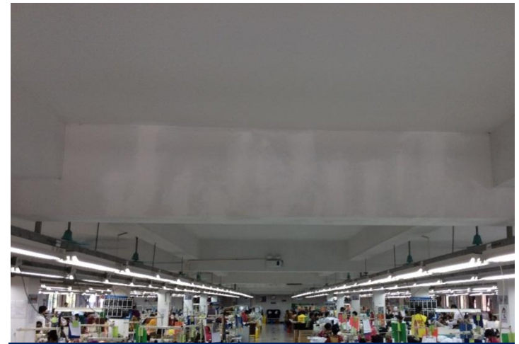
Cracks Repaired to side of the beam
