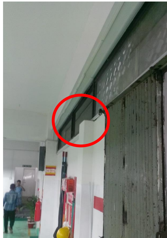
1 st floor by stairwell (Internal wall)
