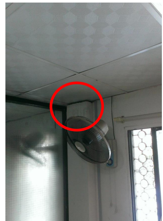
1 st floor office (External wall)
