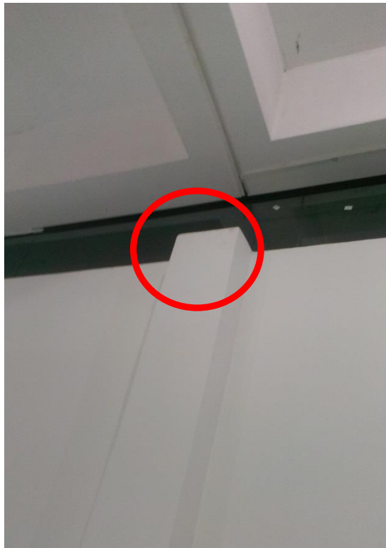
Ground floor between childcare and medical room (Internal wall)
