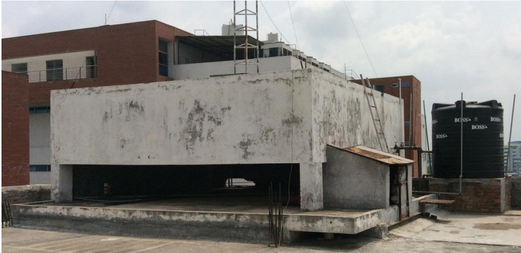
RC Tank over North East Stair Core
