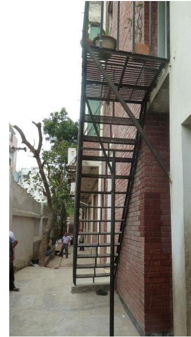
Stair to Residence
