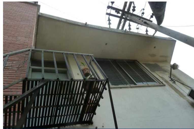
Two storey Residence and Child Care addition
