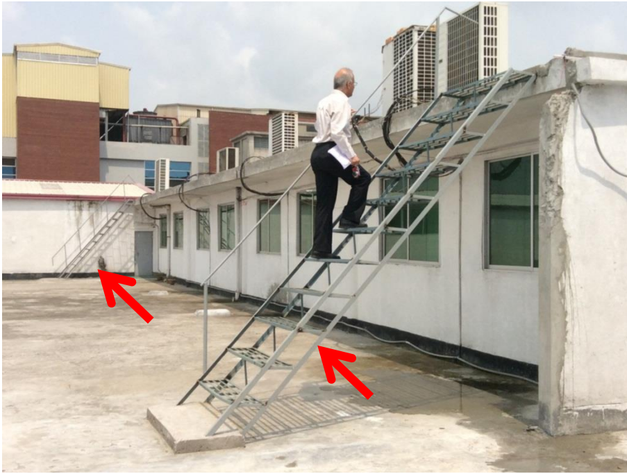
Stairs to Main Roof Slab
