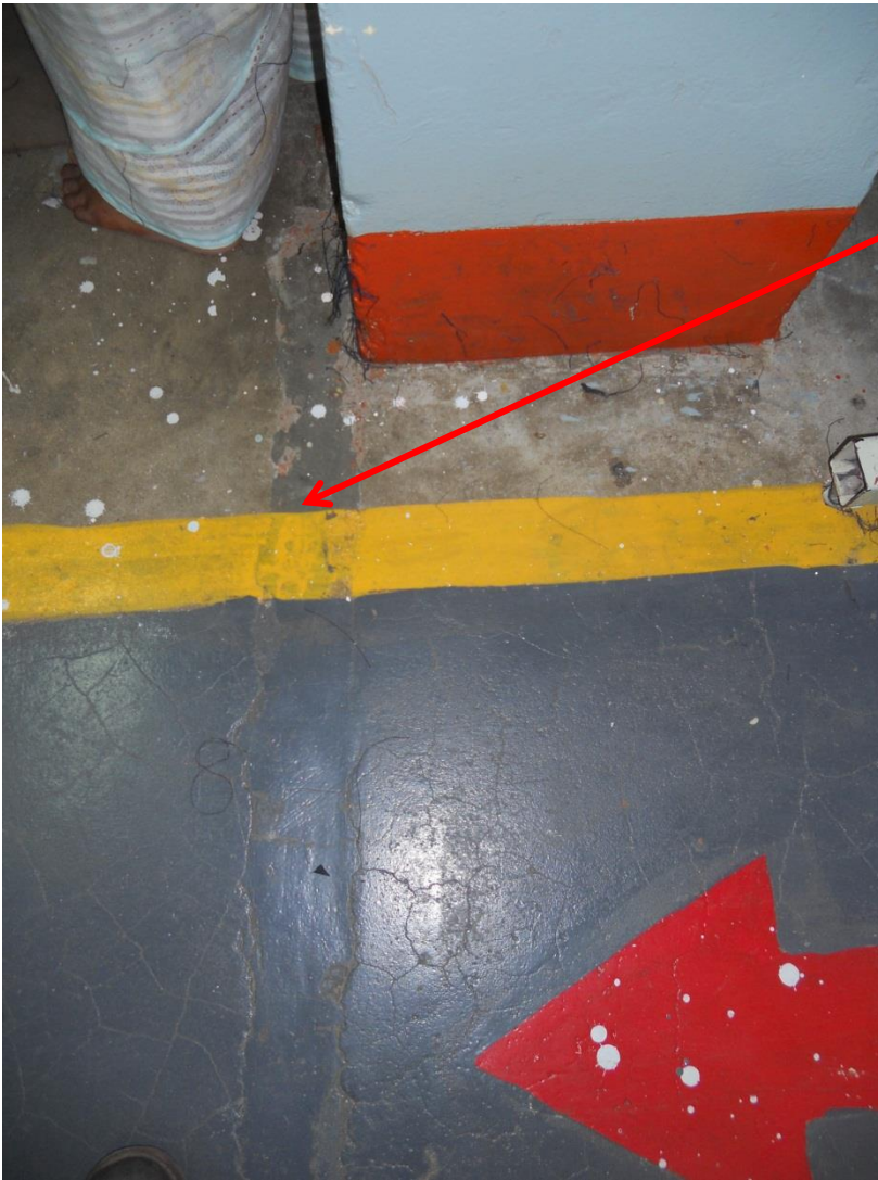
Cracking in Floor Slab Surface
