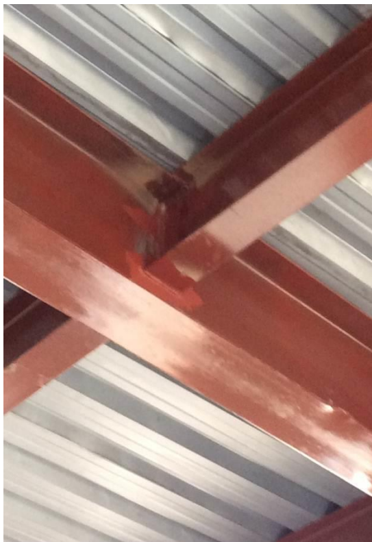
Typical Mezzanine Welded Connection
