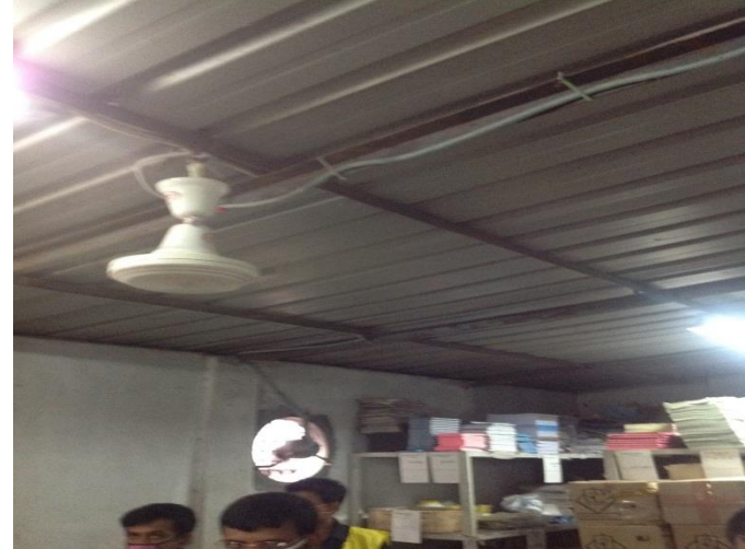
Main building office
