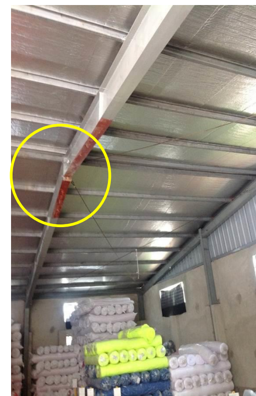
Original building extension portal moment connection
