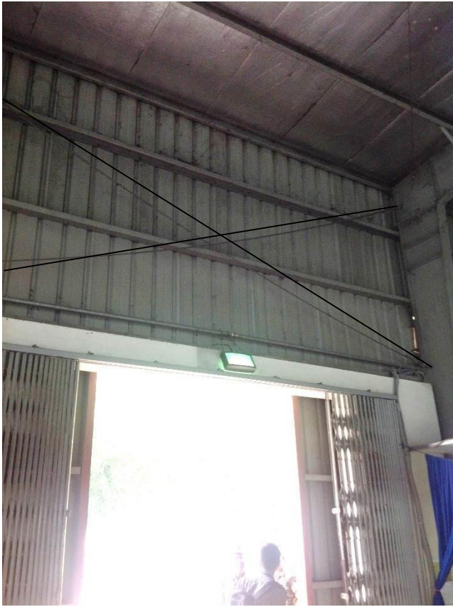
North Face Wall Bracing
