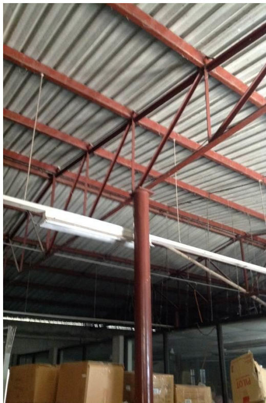
Original building truss to CHS Connection
