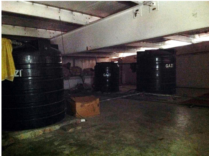
Water tank loading on shallow secondary slab above toilet areas in Building 2.
