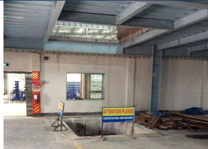
New lift pit in knitting building
