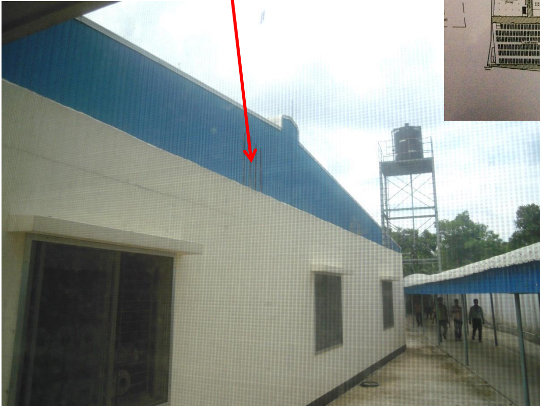
Possible future extension works noted
