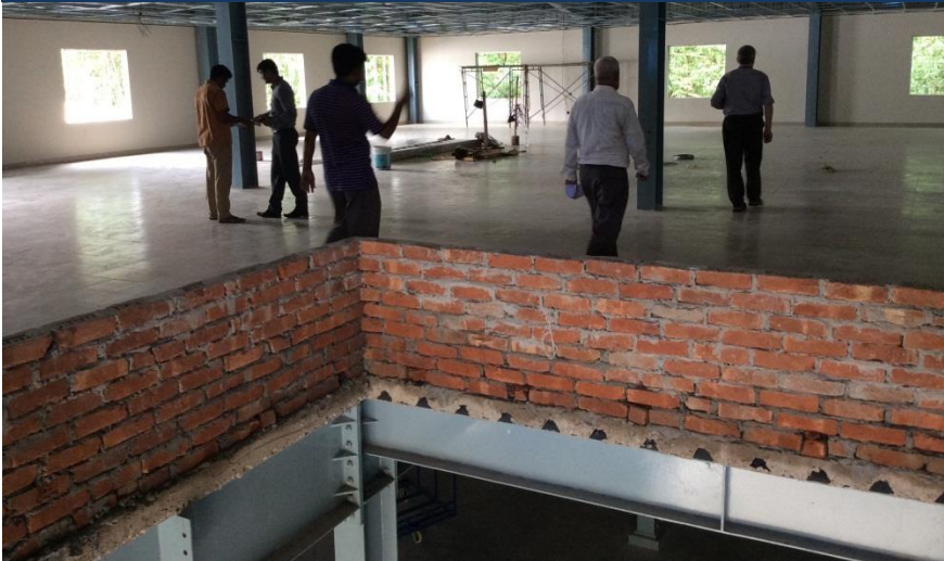
Lift pit in new warehouse building
