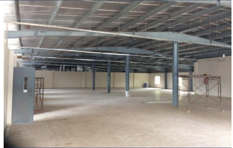
Level 01 of New Warehouse Building
