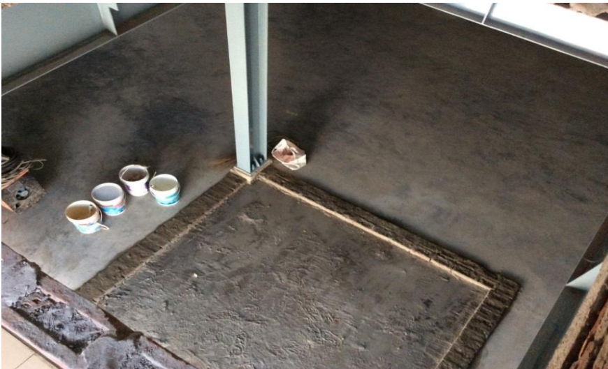
Construction works ongoing
