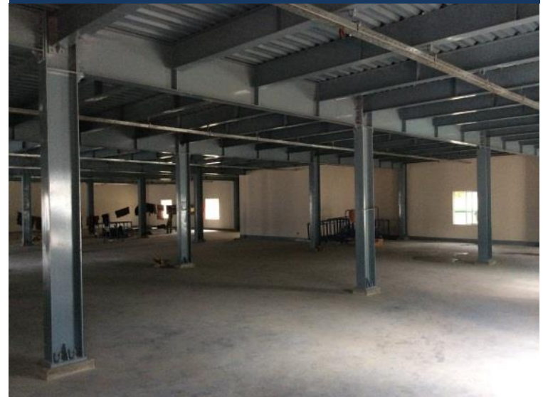
Ground Floor of New Warehouse Building
