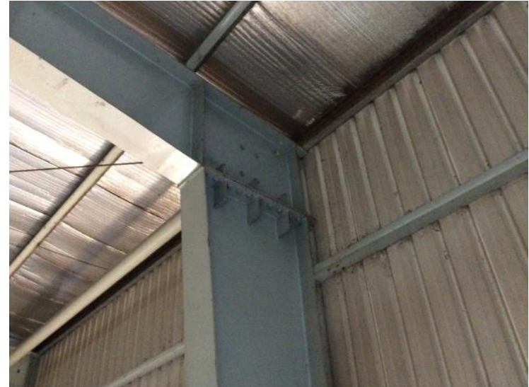
Typical portal frame steel connection
