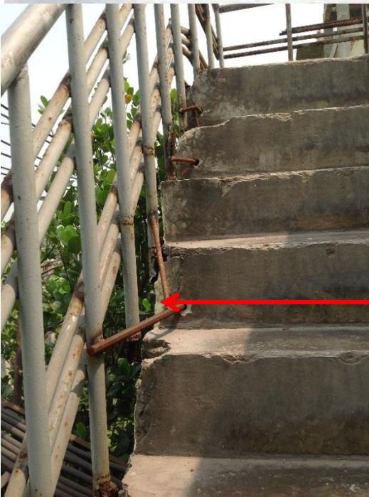
Defective Handrail
