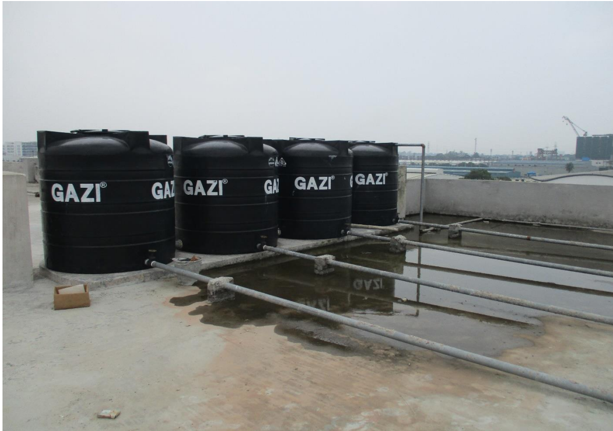
Water ponding on main factory building roof
