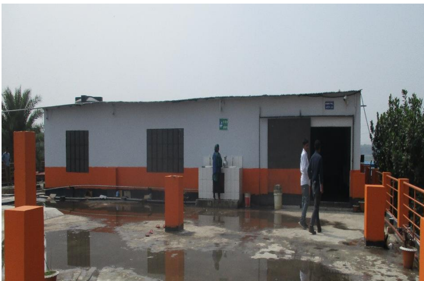
Apparently non-engineered steel shed
