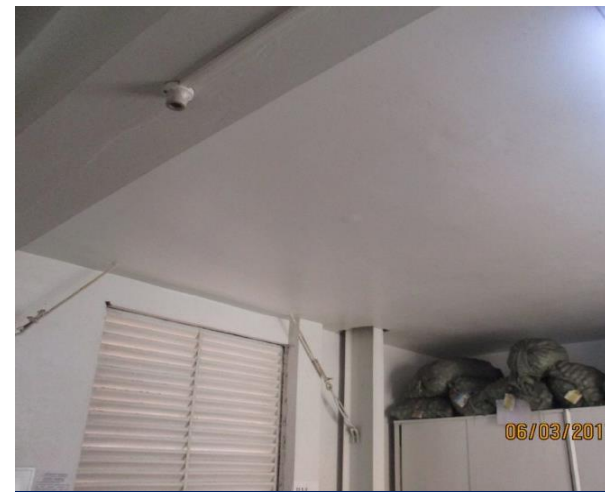
4.7m extension of RC slab supported on load bearing wall at east side.
