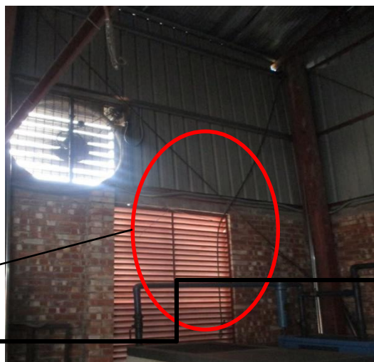
Untied vertical bracings at North side
