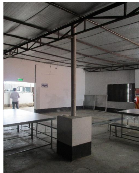
Truss to pipe connections
