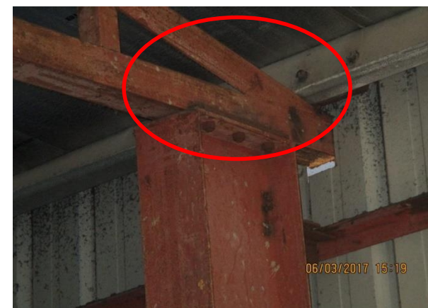
Bolted connection between steel truss and column.
